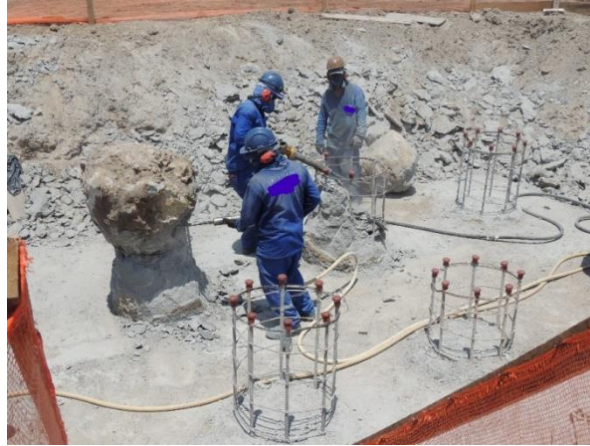
Figure no 5 - Picture of the 1st place Good practices in pile driving activity
