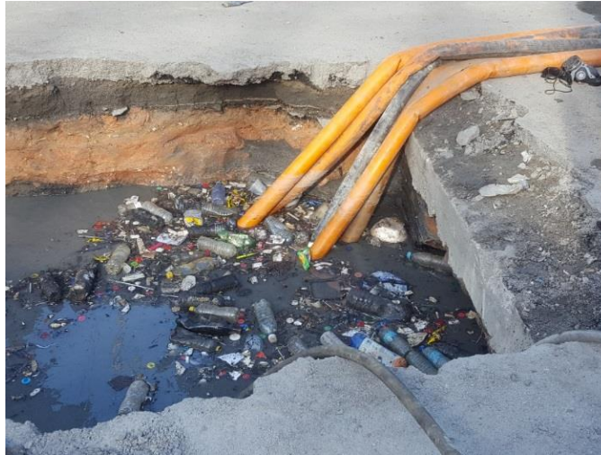
Figure No. 3: Execution of works to remove obstructions in the drainage network.
