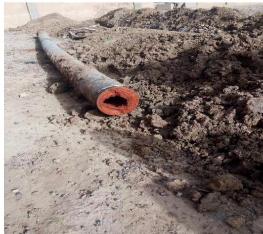
Figure No. 1: Water pipe scaled by a ferric deposit
