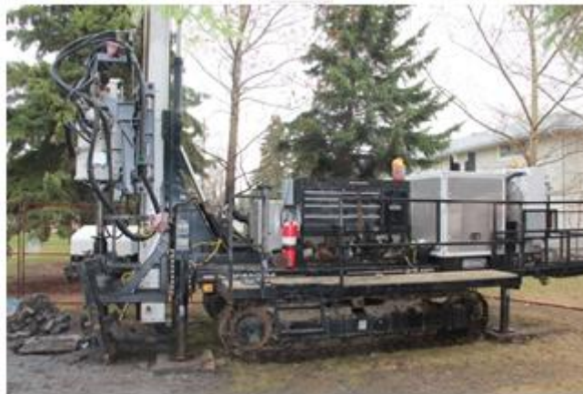
Figure 1: Drilling of the boreholes for UTES project.
