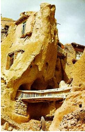
Figure 4. View of a wooden bridge.
