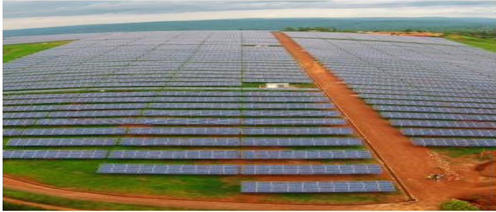
Figure 6: Gigawatt global at Rwamagana district (Republic of Rwanda, Ministry of infrastructure, 2015).
