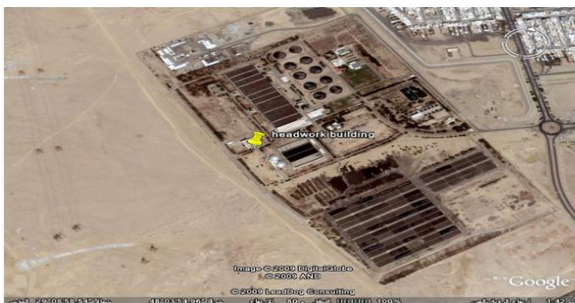
Figure (1) Riqqa Plant
