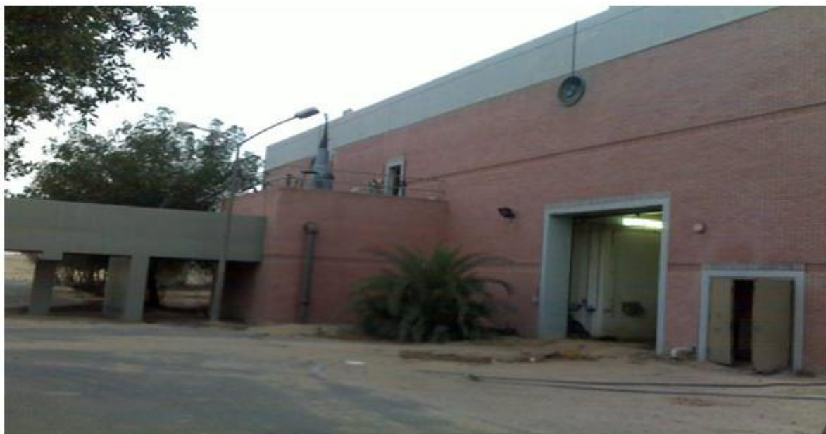
Figure (2) Photo Headwork's Building
